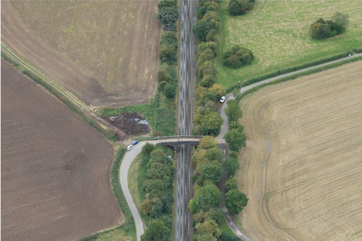
Burbage Common Road Overbridge (Existing)
